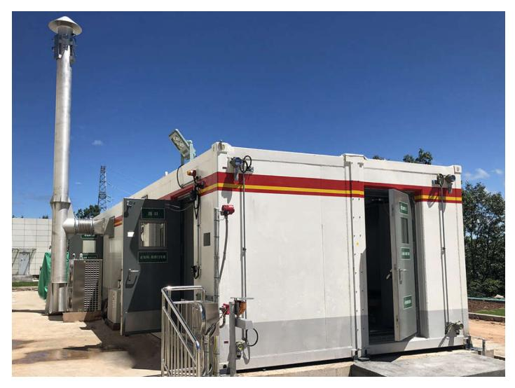
Uniteam 40-men SIP is SIL-2 certified system and is a customized solution built for easy transportion and relocation. It is built by 2 sets of 51ft containers size consisted, fire rating A-60 and blast protected 690mbar/20msec.
