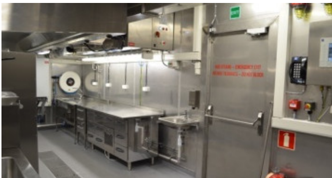
Workspace inside 32ft Kitchen Container
