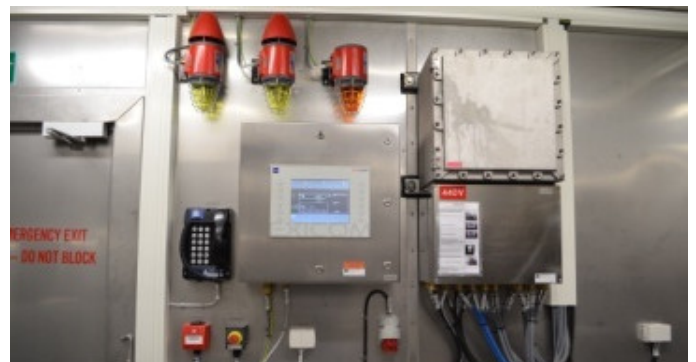
Full installation accNorsok Z-015, Type A - Galley
