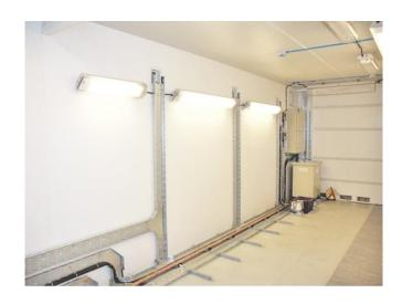
Custom-made Instrumentation Container certified according to DNV 2.7-1, manufactured in accordance with NORSOK Z-015 and special customer demands.
