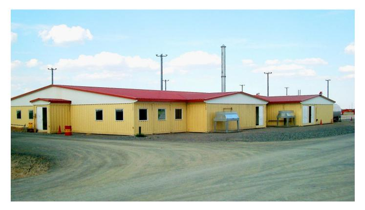
Please find below the description of this Uniteam 750 man SIP, customized solution built for easy transport and relocation as it's built by 47 standard ISO containers size (45x40' and 2x10'). The sealing between the containers solved by Uniteam patented GSSP gaskets, gives quickly deployment of SIP at site, with minimum downtime of the ongoing production.
