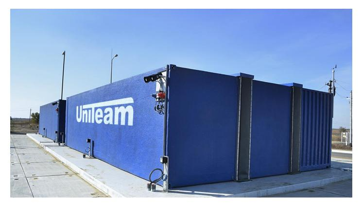
This Uniteam 50-men SIP is GOST-K and SIL-3 certified and is a customized solution built for easy transport and relocation. It is built by 4 standard ISO containers size (2x40' and 2x20') fire rating A-60/J-45 (Jet-fire protected) and blast protected to 200mbar/45msec. The sealing between the containers is solved by Uniteam patented GSSP gaskets which ensures fast deployment of the SIP on site, with minimum downtime of the ongoing production.
