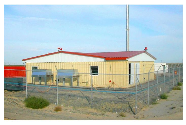
Please find below the description of this Uniteam 250 man SIP, customized solution built for easy transport and relocation as it's built by 11 standard ISO containers size (10x40' and 1x10'). The sealing between the containers solved by Uniteam patented GSSP gaskets, gives quickly deployment of SIP at site, with minimum downtime of the ongoing production.
